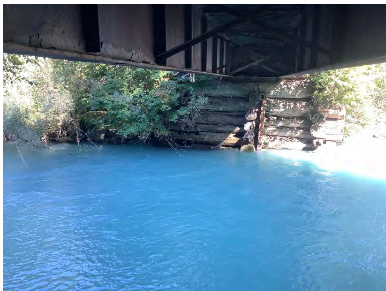
Left Bank Abutment when facing downstream
